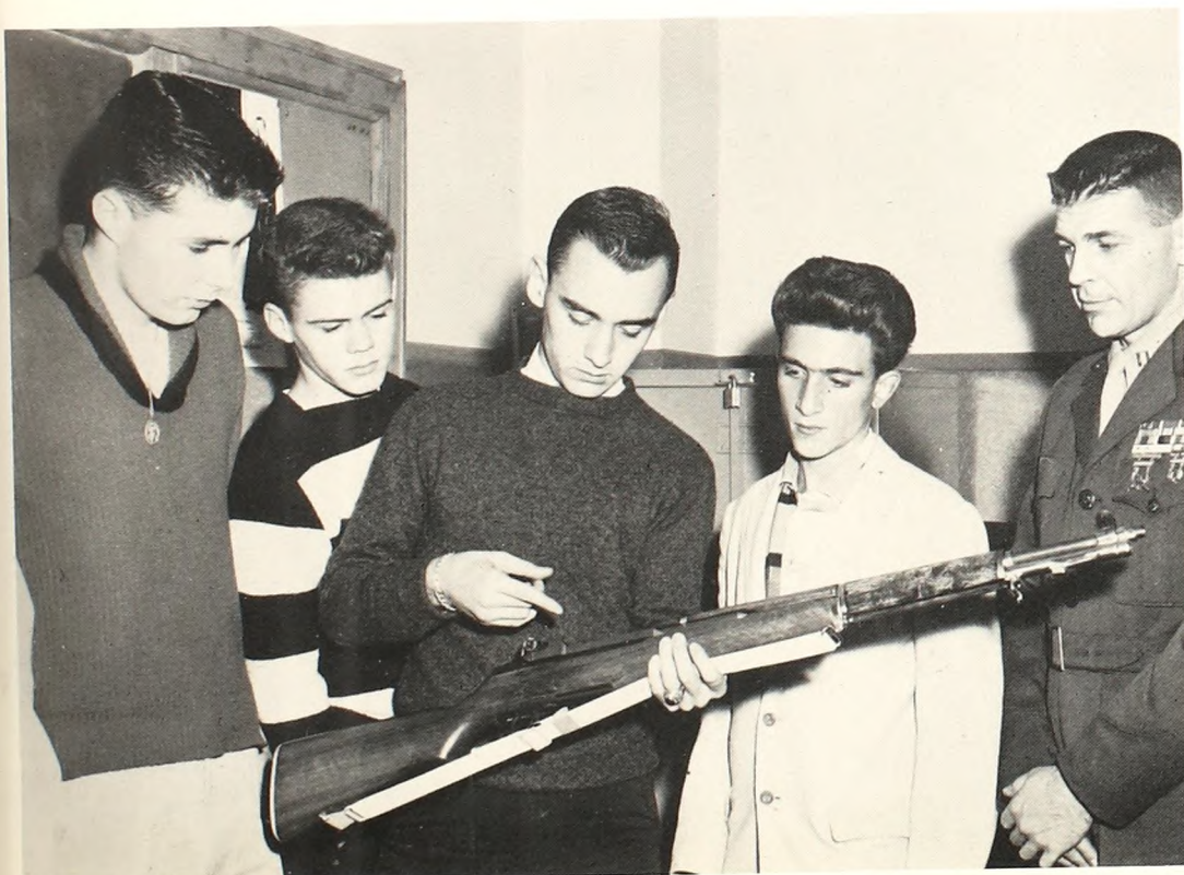
One of the many lectures dealt with the working of the M-1 rifle. Here, a Corps representative begins to reassemble the weapon.
